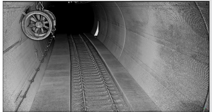
grey-scaled point cloud of subway tunnel
